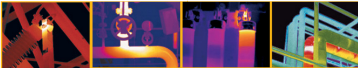
Fig. 3 – Thermal imager application for various industrial system troubleshooting [4]
